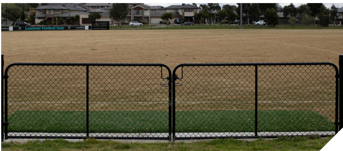
Double gate access to the playing field to enable emergency vehicle and/or curator machinery easy entry/egress.
